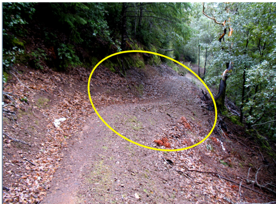
Photo 6.7 - Using a Drain Dip to Divert Water Off of the Trail
