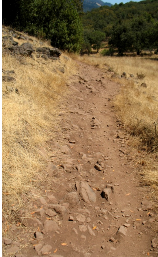
Photo 6.6 - Using Native Rocks to Texture Surface and Reduce Speed
